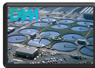
UC5: Critical wastewater treatment decision support enhanced by distributed, AI enhanced edge and cloud solutions
